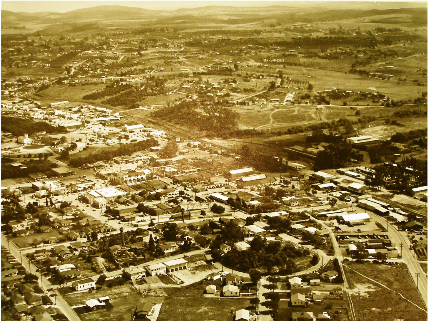
Vista 1953 looking south from The Circle
