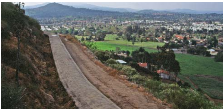
Cover photos: VID Flume - Local Water Transportation Structure Top: Picture of the Flume being constructed in the 1920's Bottom: Picture of the modern day completed Flume
