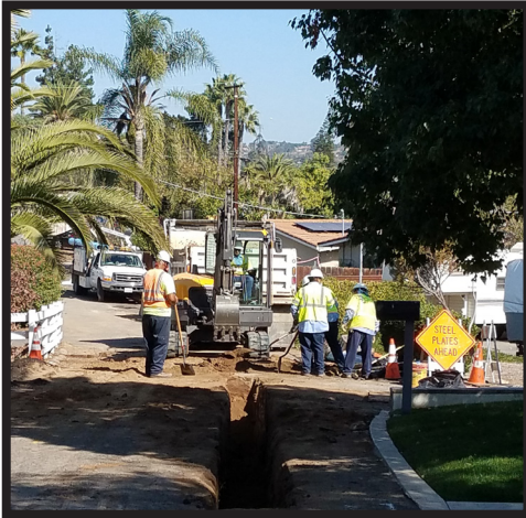
Pictured: Mainline Replacement on Rosario in Vista
