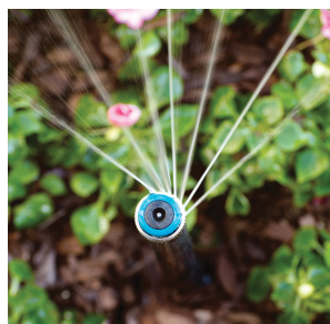
Rotating Sprinkler Nozzle Rebates
