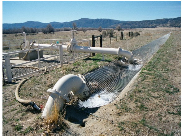
Figure 2. Groundwater Wells Discharging to Ditch at Location 1 on the Warner Ranch.
