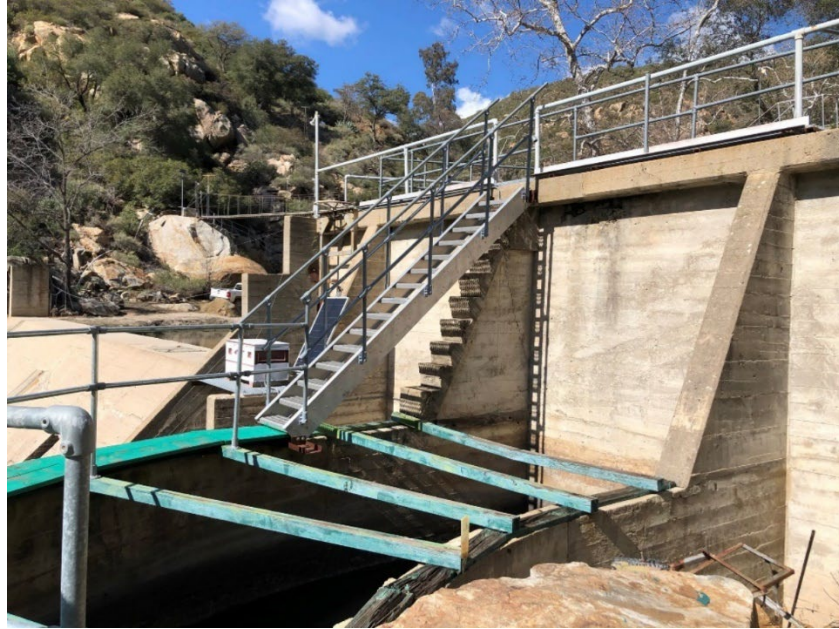
Figure 2-32. Escondido Canal Diversion Dam looking upstream from the right bank, March 4, 2021.
