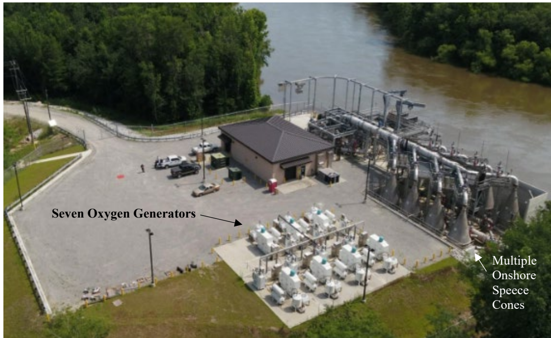
Figure 4-14. Example oxygenation system with onshore Speece cones and oxygen generators. Photo Reprinted from US Army Corps of Engineers Startup Run Data Collection & Modeling Report , Oxygen Injection System Environmental Testing for the Savannah Harbor Expansion Project, March 2021.
