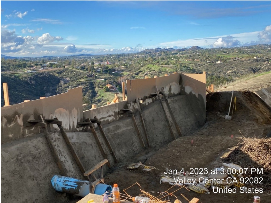
Pumping shotcrete for the gravity wall
