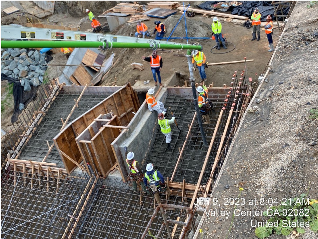
130 yards of concrete pumped for half of the slabs on Monday 1/9/23.
