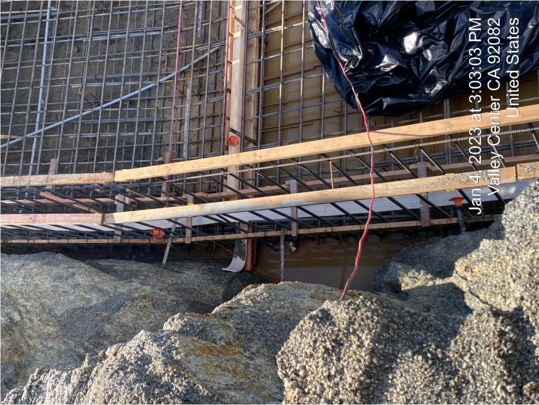
Recent rain's impact on the desilting basin
