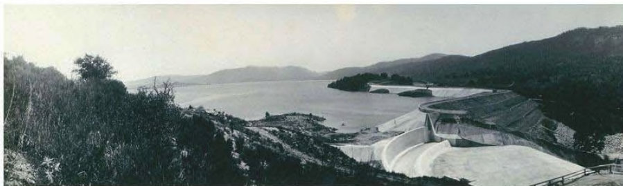
Henshaw Dam April 5, 1928
