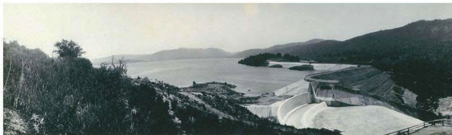
Henshaw Dam April 5, 1928
