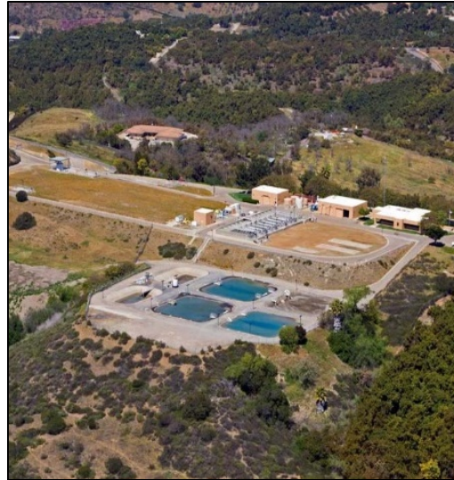
Oceanside and VID Interconnects
