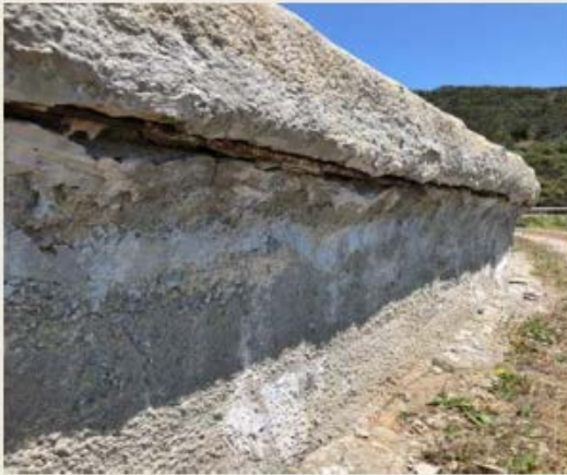
Not suitable for reuse. Left : Roof separation, Borden Bench; Right : Erosion under Daley Bench
