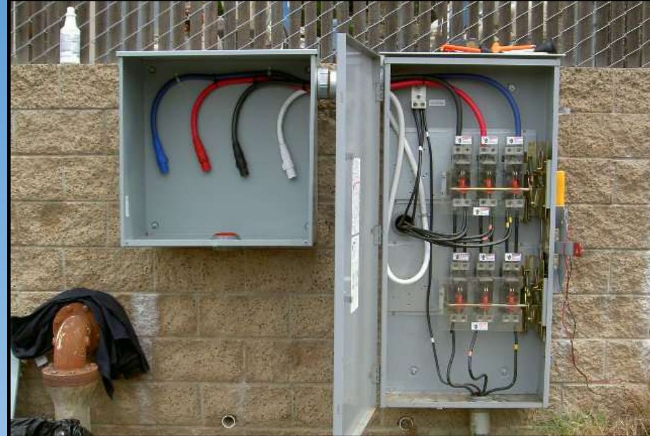
Pump station transfer switch/generator connectors
