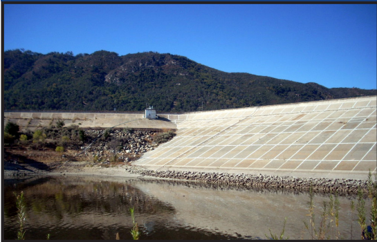
Henshaw Dam is re-engineered for seismic reasons, reducing the lake's capacity from 200,000 acre feet to 50,000 acre feet.
