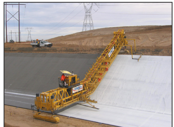
All American Canal Paving Photo Credit: Water Authority
