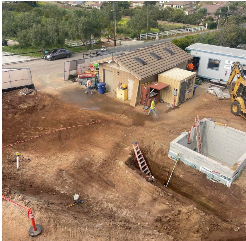
Export Excess Soil (Above) Begin Yard Piping Excavation (Below)
