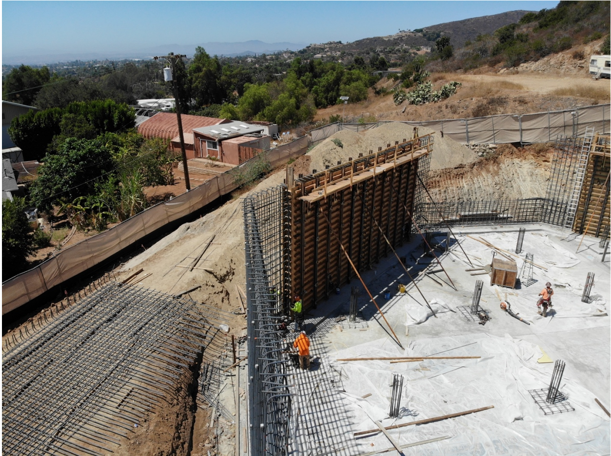
Preparing wall rebar at and forms (Above)
