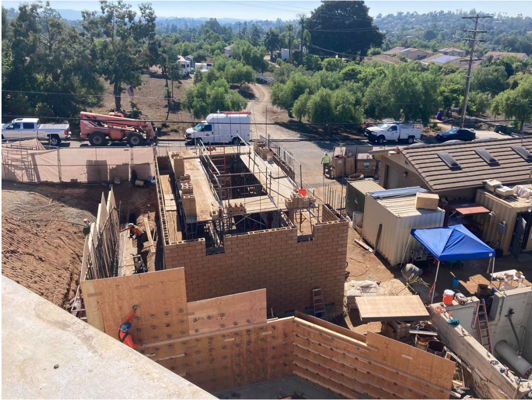
Pump Station CMU Block and Retaining Wall
