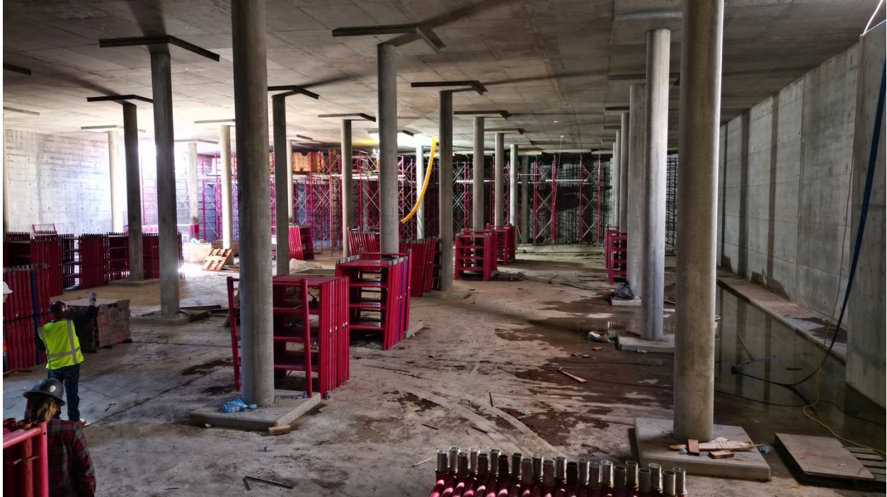
Roof Deck Shoring Removal (above). Roof Deck Shoring Remaining Until Concrete Reaches Strength (below)
