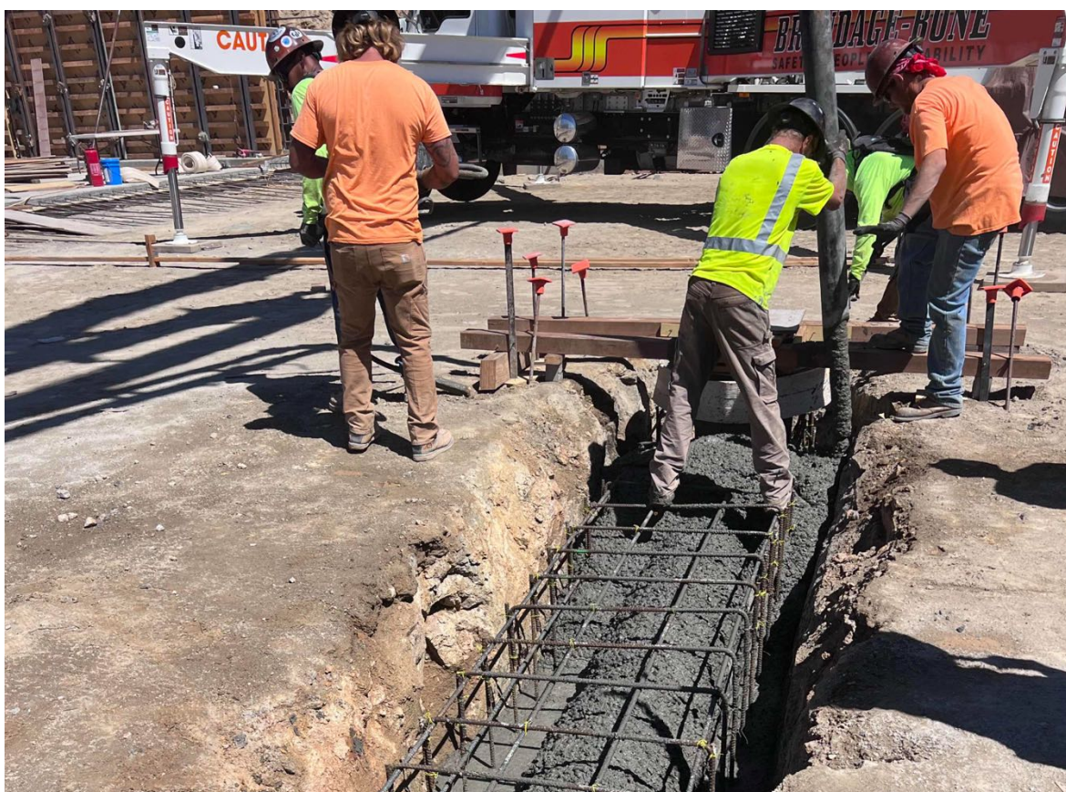
Outlet pipe installation and encasement
