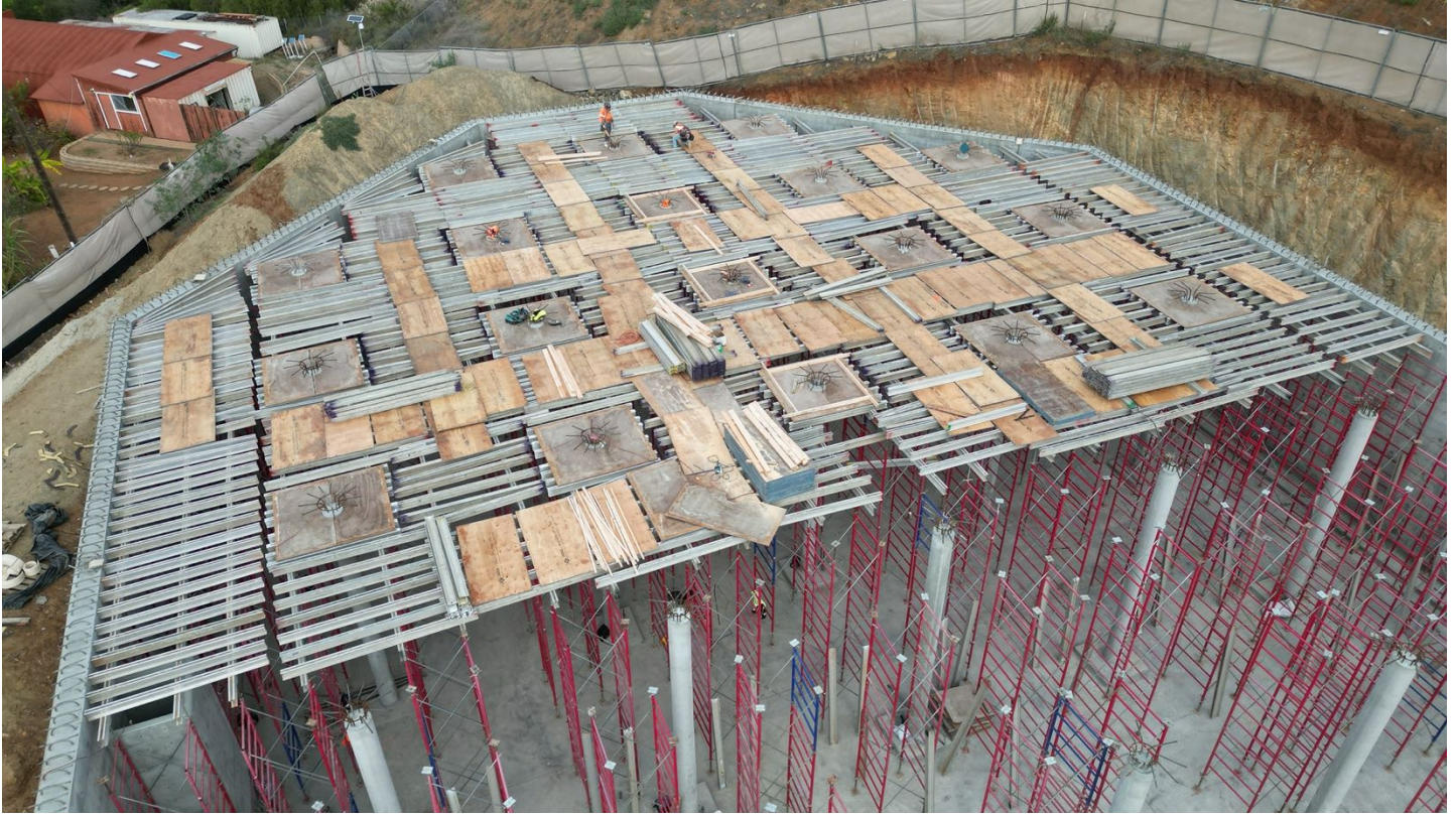
Roof Deck Shoring Installation and Decking Installation
