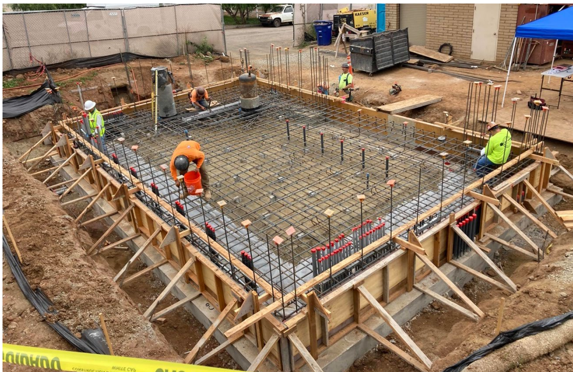
Pump Station Slab Electrical Conduits (Above) Pump Station Slab Rebar (Below)
