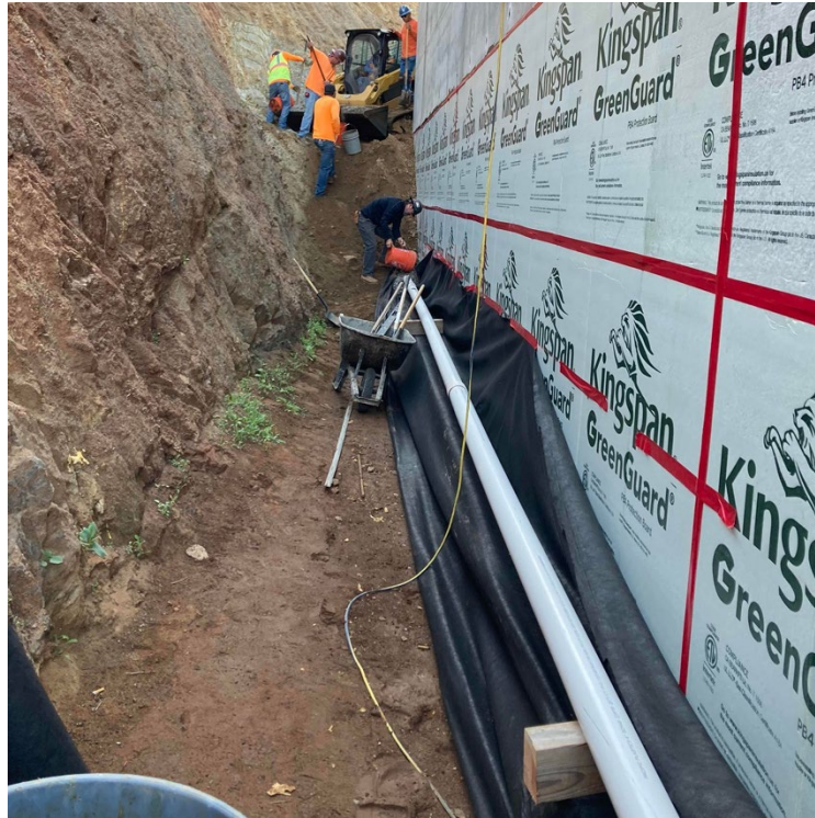
Reservoir Footing Drain/Backfilling (Above) Pump Station Retaining Wall Footing (Below)
