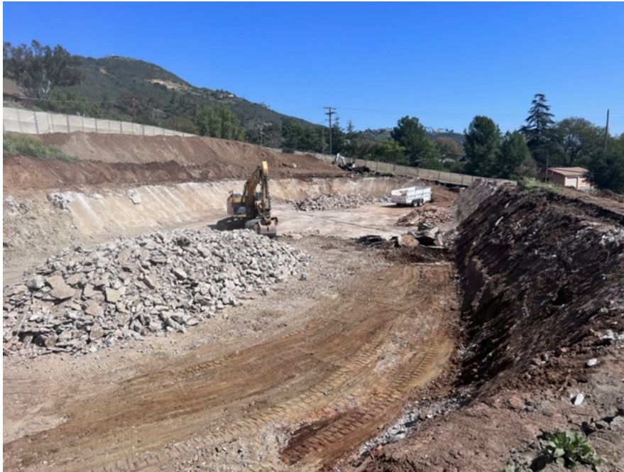
Removal concrete reservoir walls and floor (Above)
