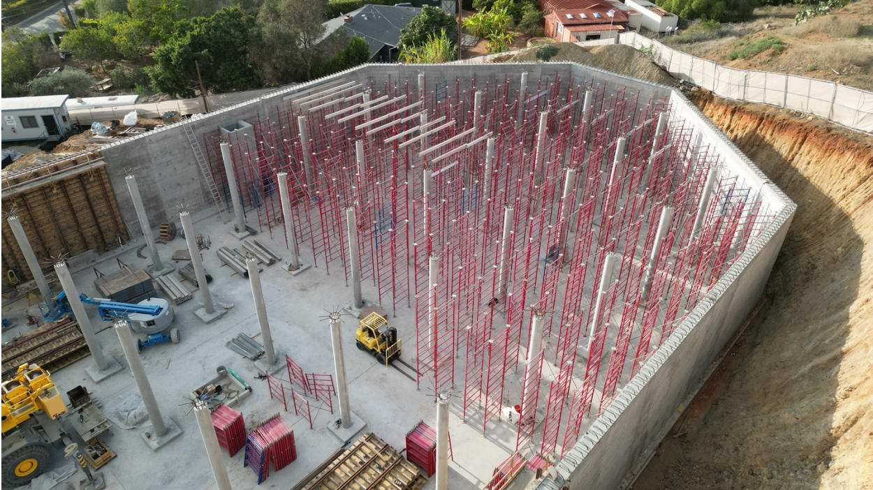
Roof Deck Shoring Installation
