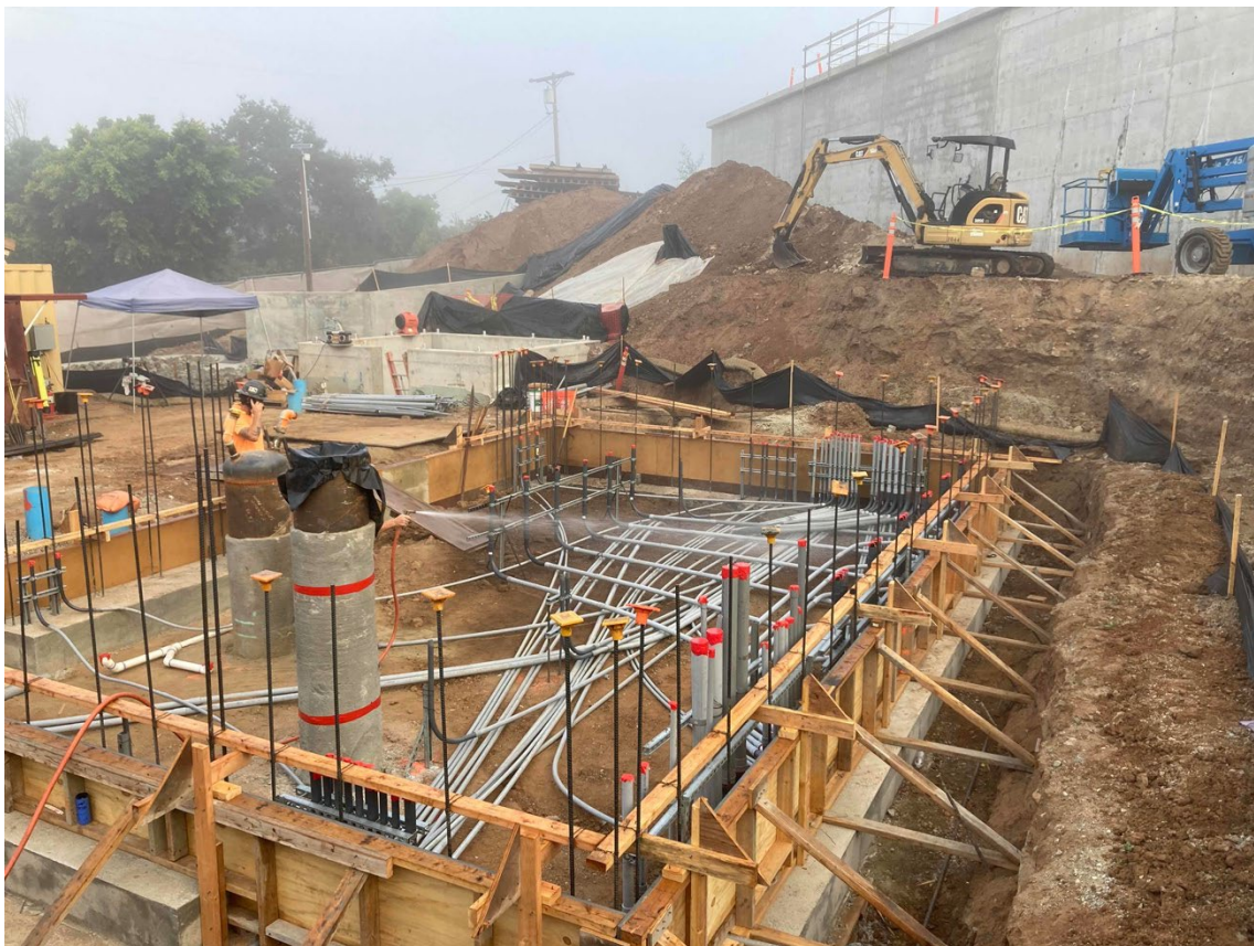
Pump Station Slab Electrical Conduits (Above) Pump Station Slab Rebar (Below)
