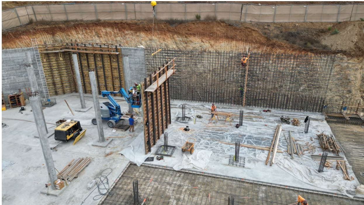
Forming of east center wall
