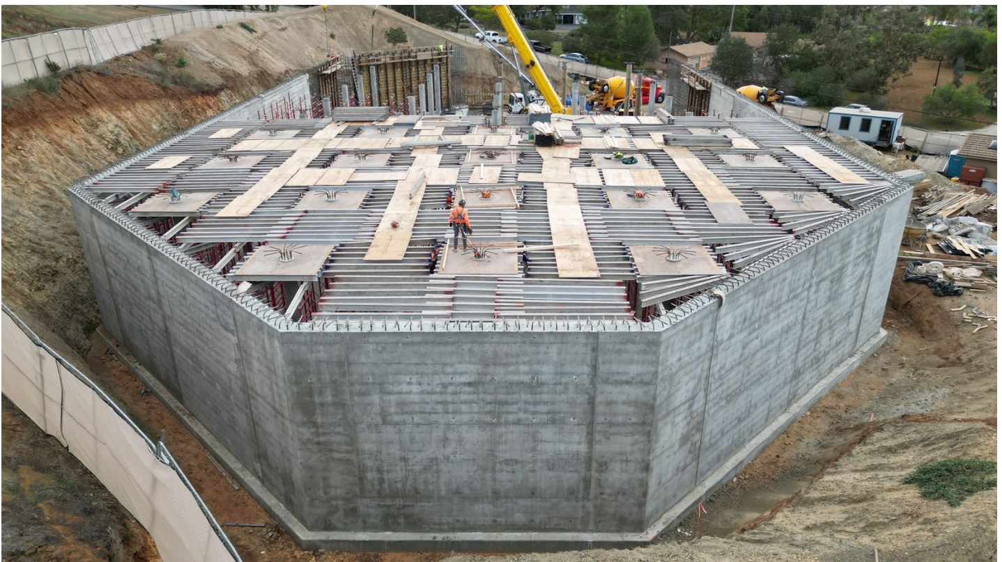
Roof Deck Shoring Installation and Decking Installation
