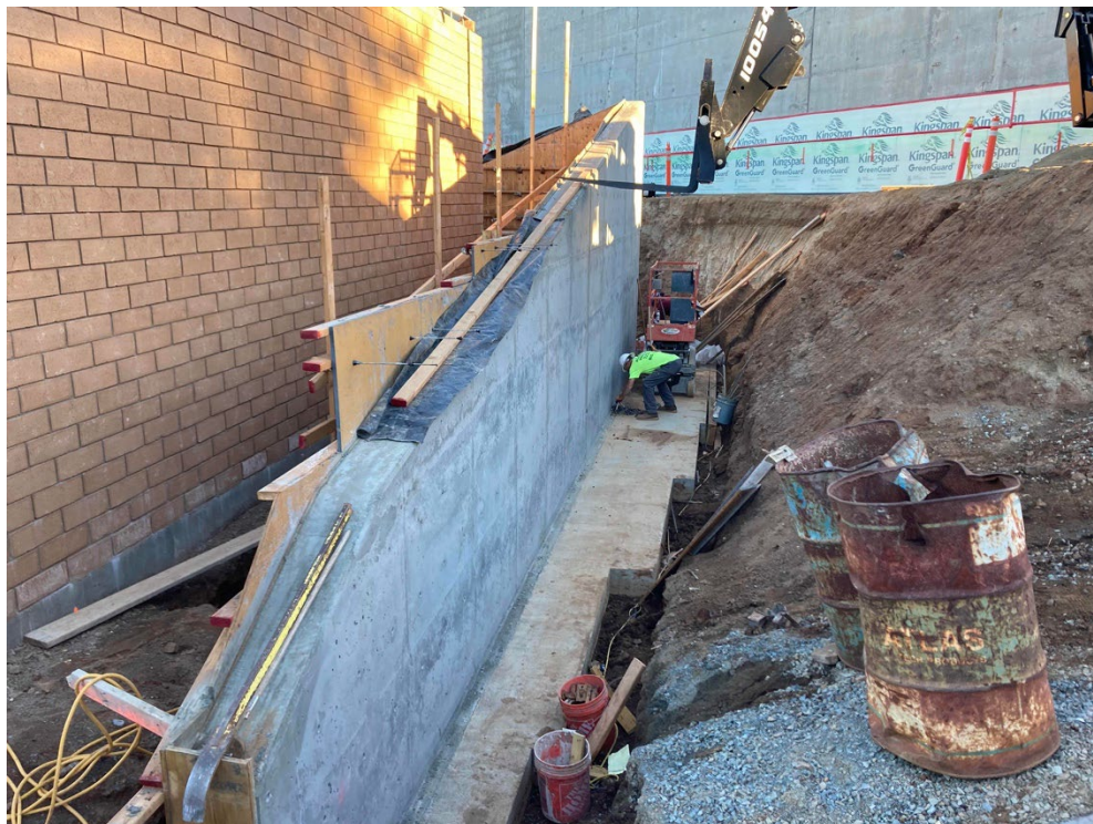
Pump Station Retaining Wall (Above) Reservoir Backfilling (Below)
