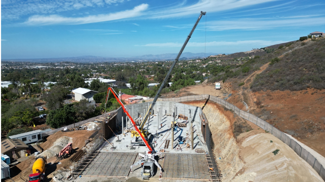
Concrete wall placement (above). Concrete slab placement (below)
