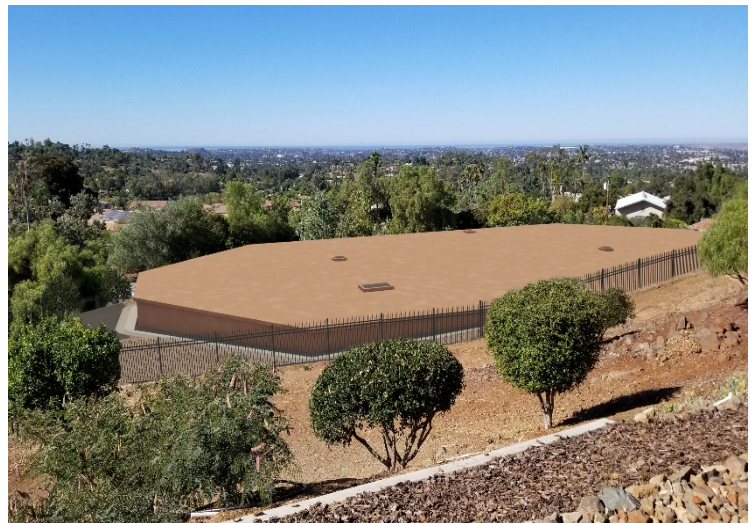
Rendering (above) of the completed project
