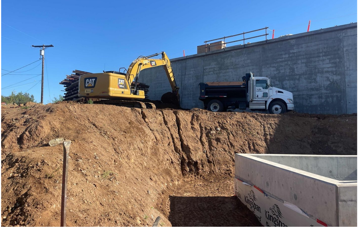
Export Excess Soil (Above) Begin Yard Piping Excavation (Below)
