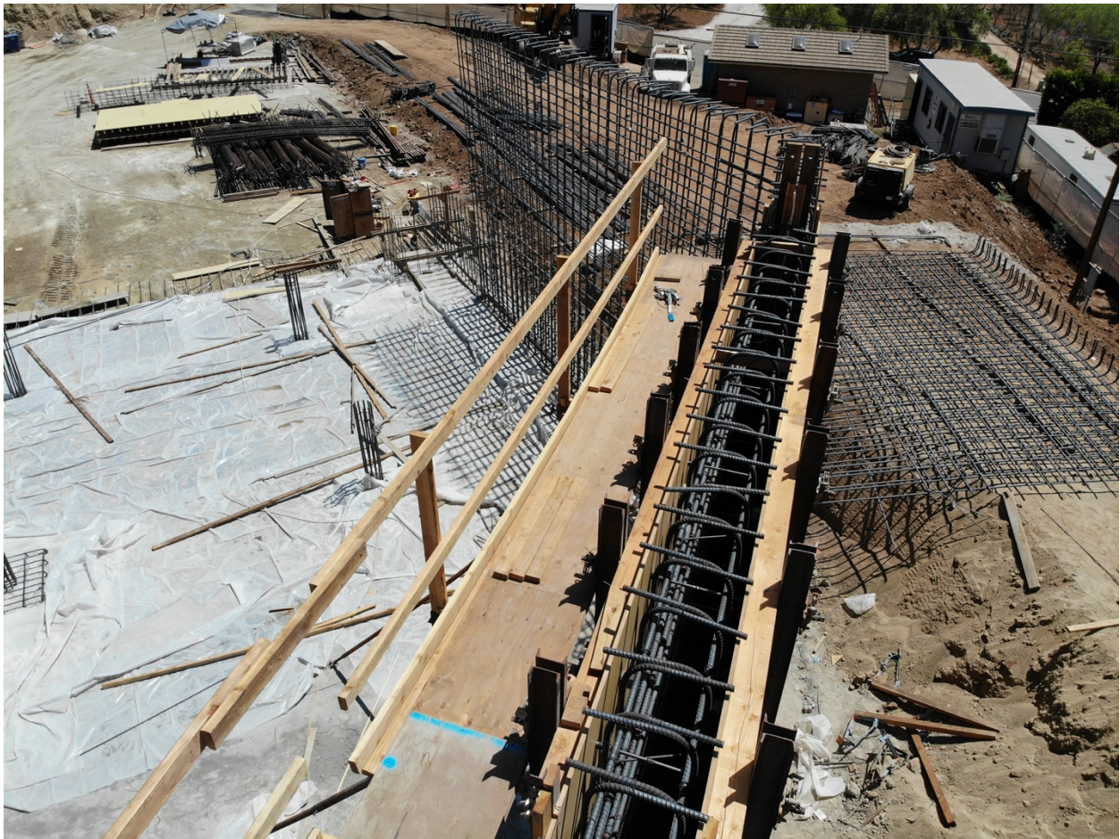
Top of Wall Forms and Rebar (Above)
