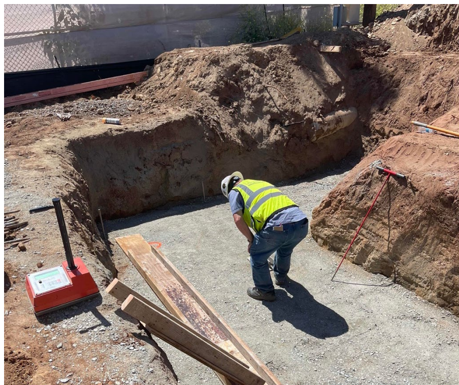
Valve Vault Valve Installation (Above) Retaining Wall Footing Compaction Test (Below)
