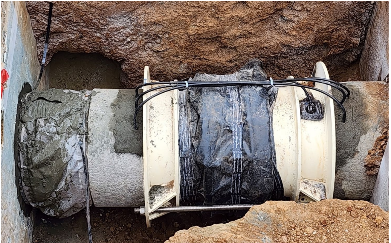
Flex Coupler Installation
