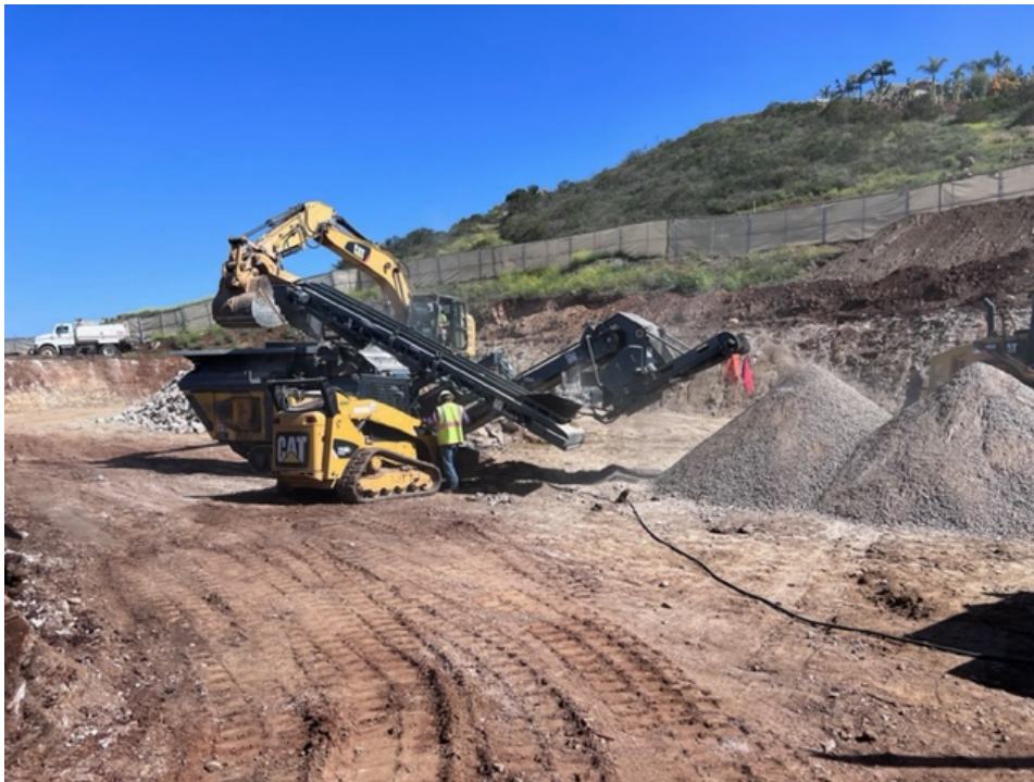
Separating concrete from steel and grinding concrete (Below)
