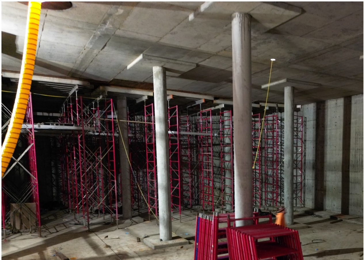
Roof Deck Shoring Removal (above). Roof Deck Shoring Remaining Until Concrete Reaches Strength (below)
