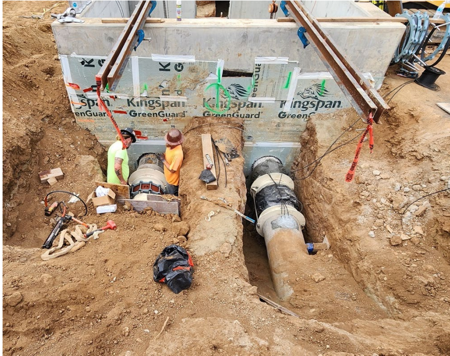
Flex Coupler Installation
