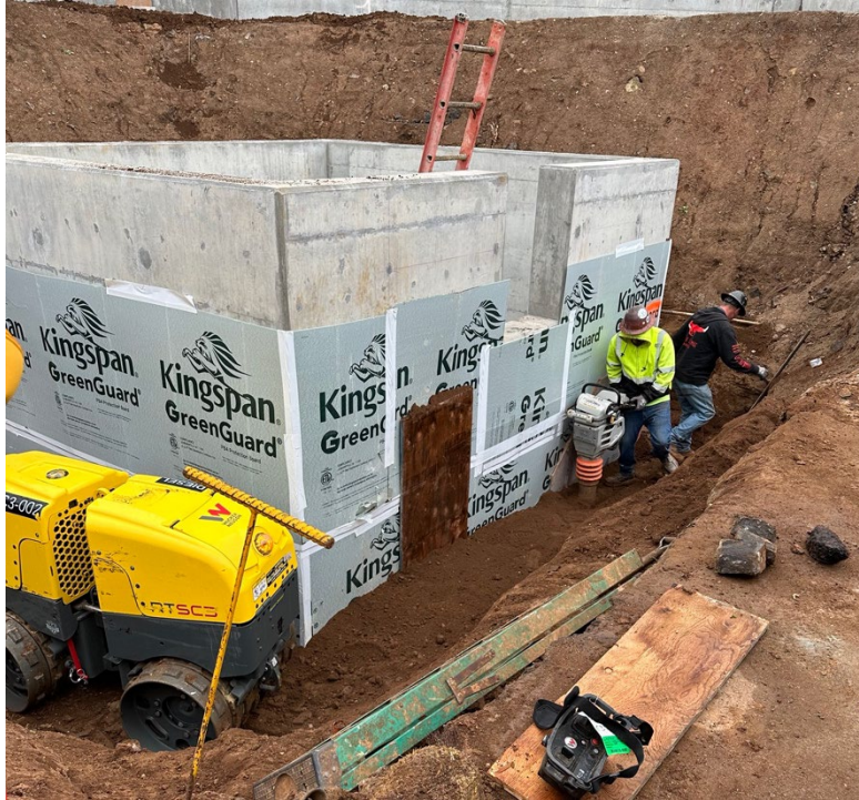
Vault Backfill/Compaction (Above) Sack & Patch Interior Reservoir (Below)
