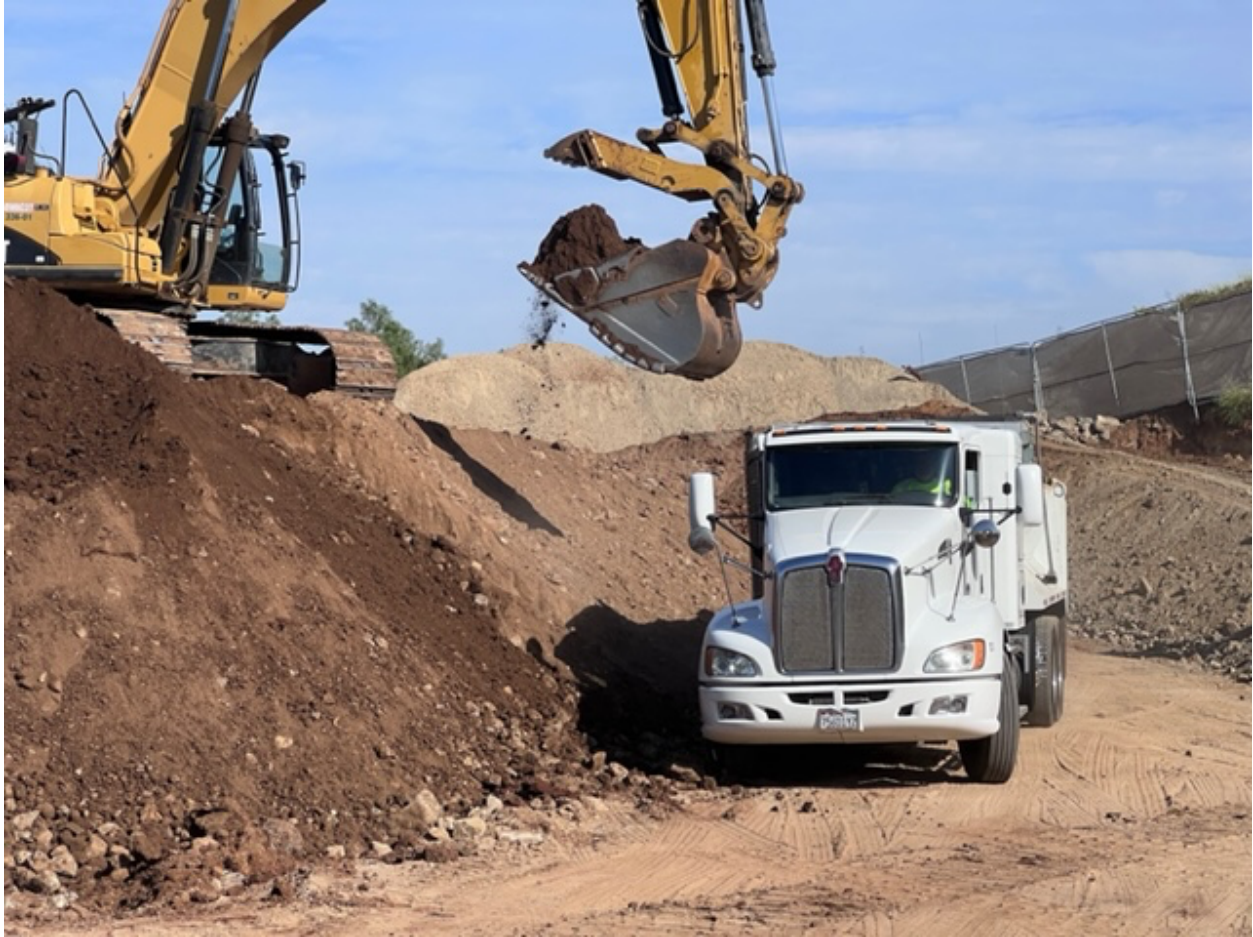
Exporting excess materials (Below)
