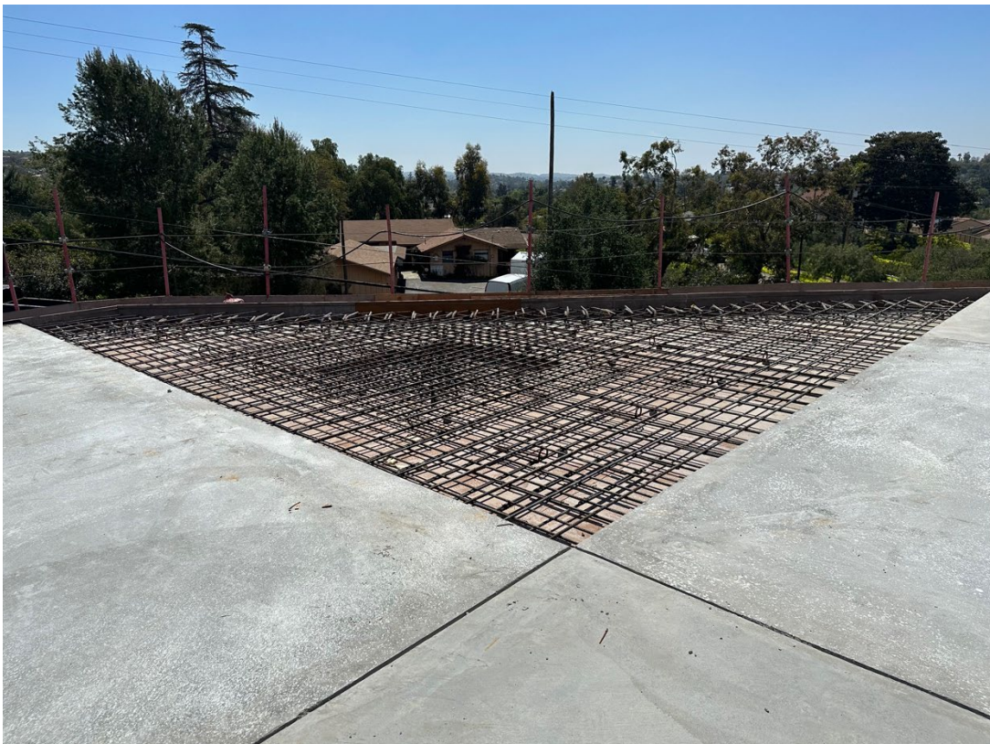
Vault Walls Formed (Above) Final roof deck pour corner (Below)
