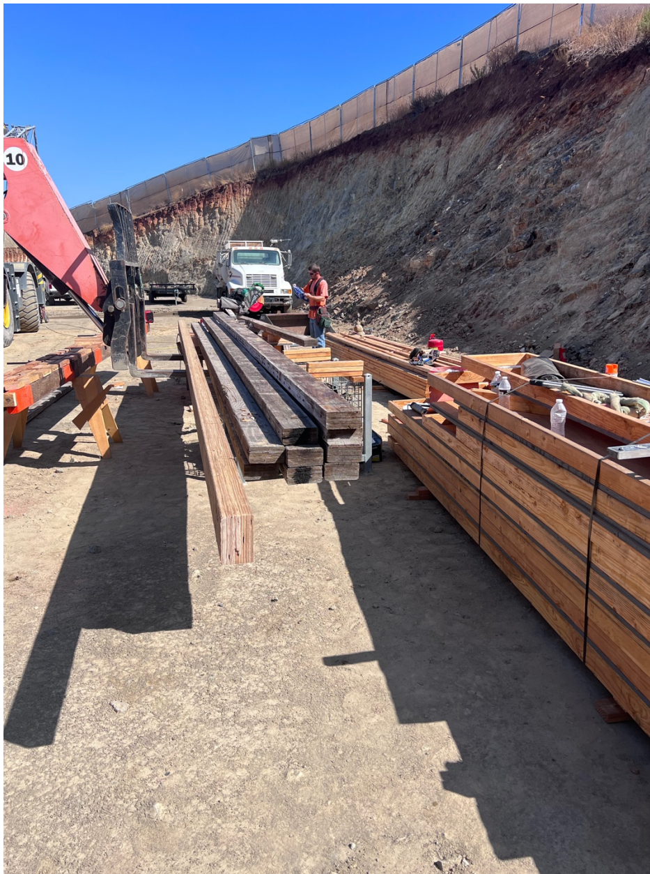
Preparing to construct edge forms (Above)
