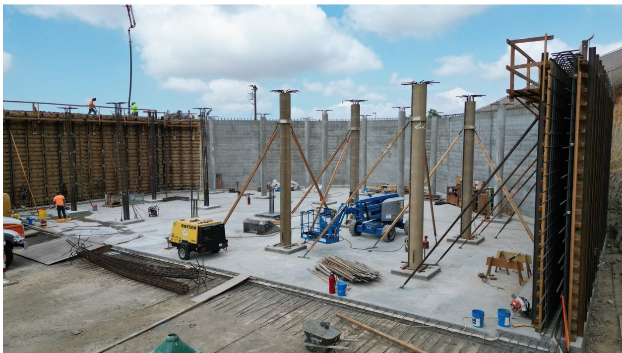
Concrete placement on west wall (above). East wall formed (below)
