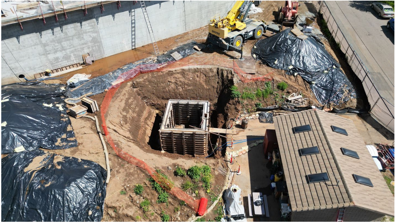
Vault Walls Formed (Above) Final roof deck pour corner (Below)
