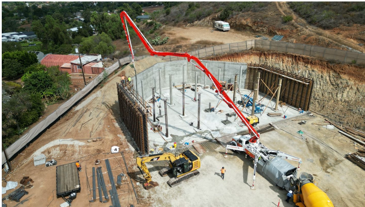
Concrete placement on west wall (above). East wall formed (below)
