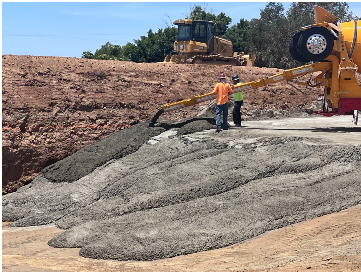
CLSM Placement (Above)
