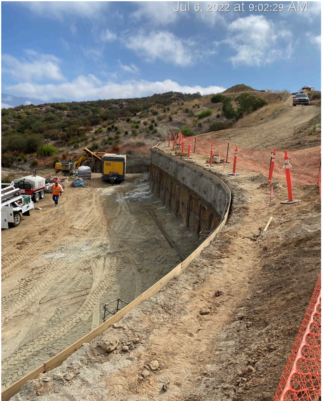
Soil nail retaining wall (seen from above).
