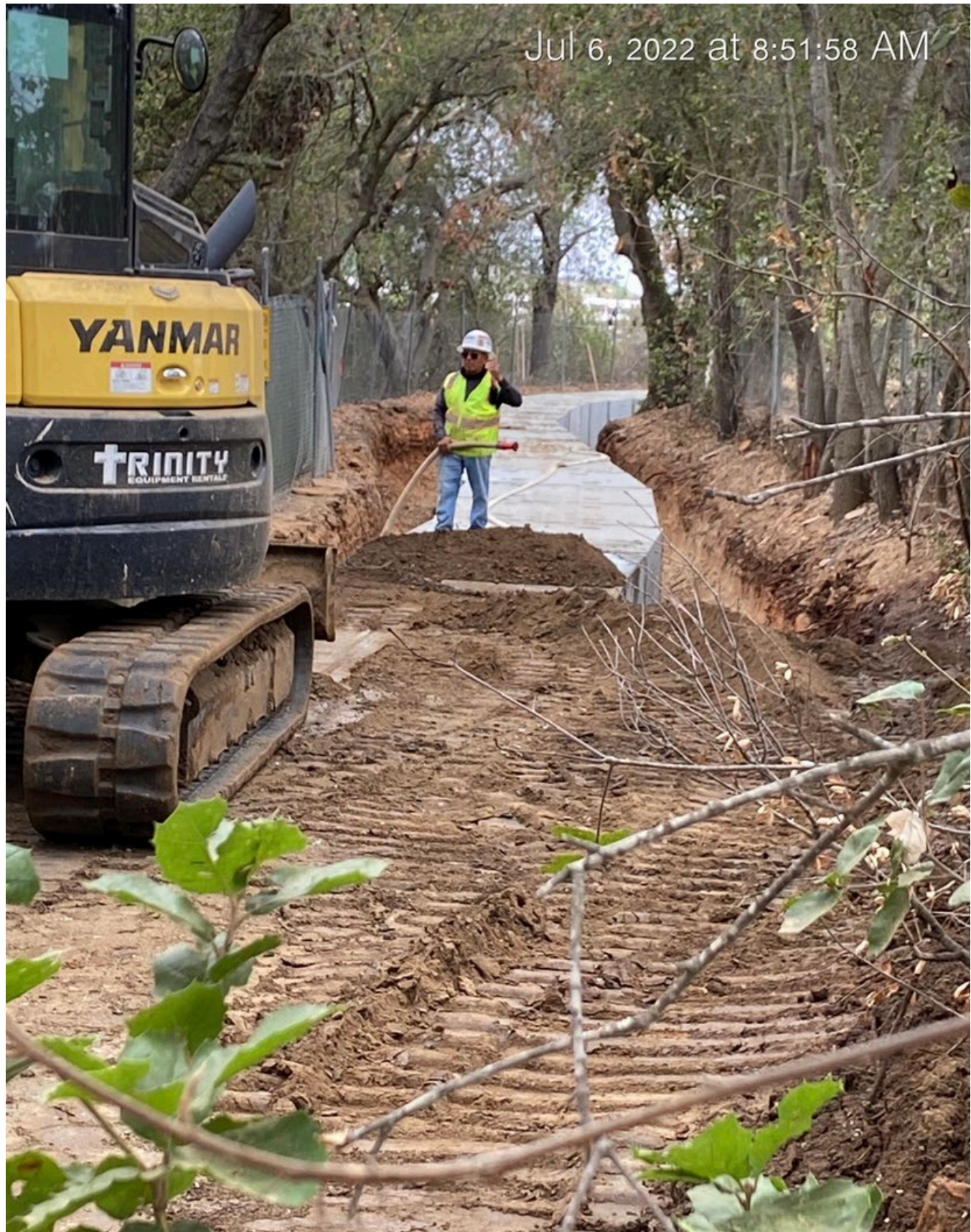
Backfill of box culvert in “Replace-in-Place” portion of project.
