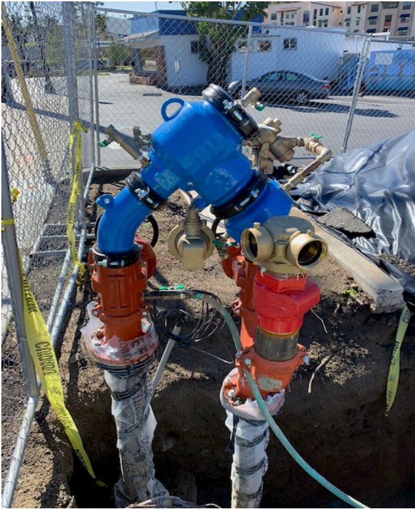
Illegal connection leading to y-fitting with additional hoses connected at 170 Eucalyptus February 6, 2019
