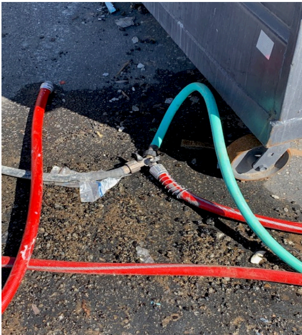
Illegal connection leading to y-fitting with additional hoses connected at 170 Eucalyptus February 6, 2019
