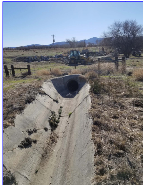
STA. 1+72.7 SIPHON OUTLET TO EXISTING CONCRETE V-DITCH.
