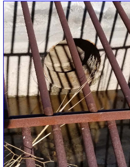
STA. 0+00 INLET TO 24" (~23.5" I.D.) CONCRETE SIPHON.
