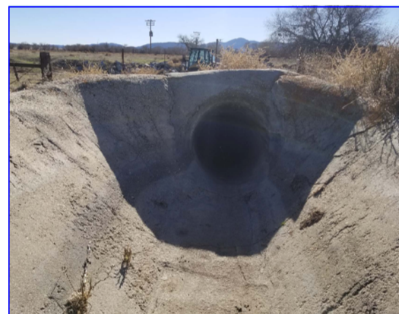
STA. 1+72.7 SIPHON OUTLET TO EXISTING CONCRETE V-DITCH (2).
