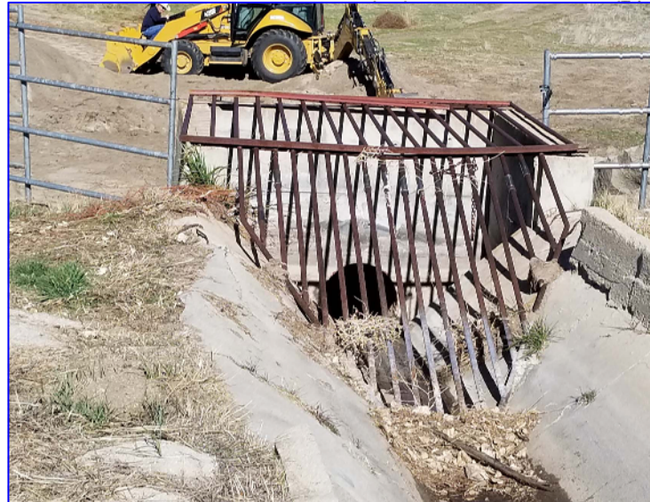
STA. 0+00 CONCRETE INLET TRANSITION STRUCTURE.
