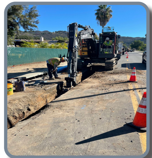
Pictured: Mainline Replacement on San Clemente Ave
