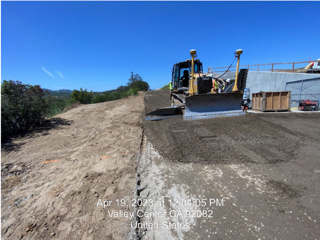
Placing Class II base on access Road
