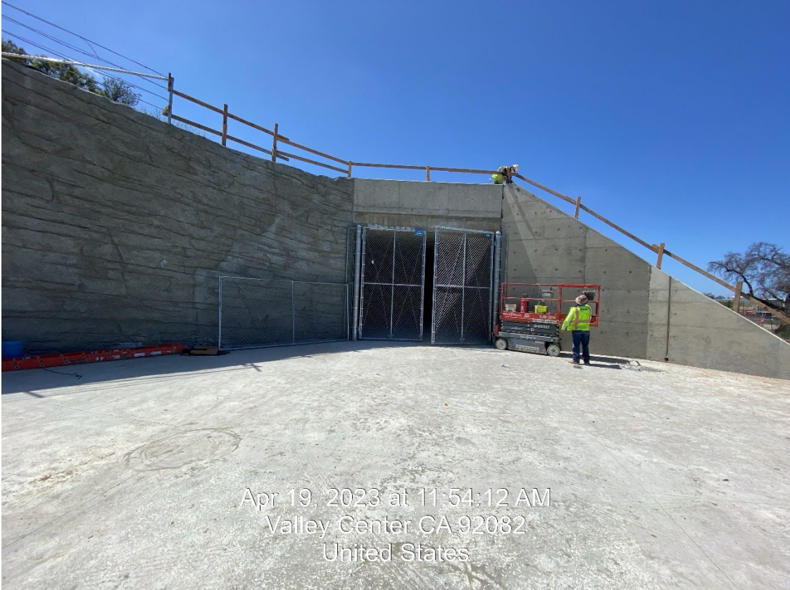
Tunnel security gate
