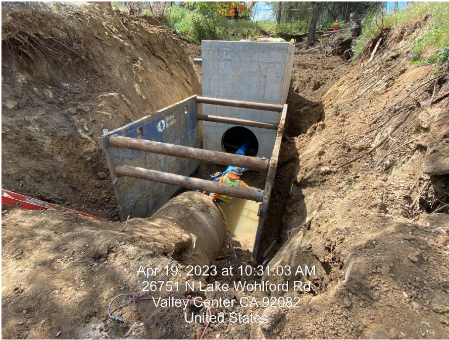
Junction structure at north and south end of CMLC pipe
