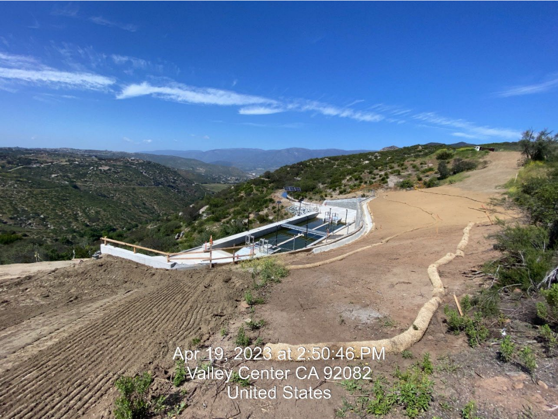
View of the basin from tunnel roof
